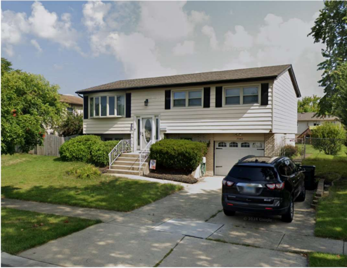
Prior to construction (July 2024)
